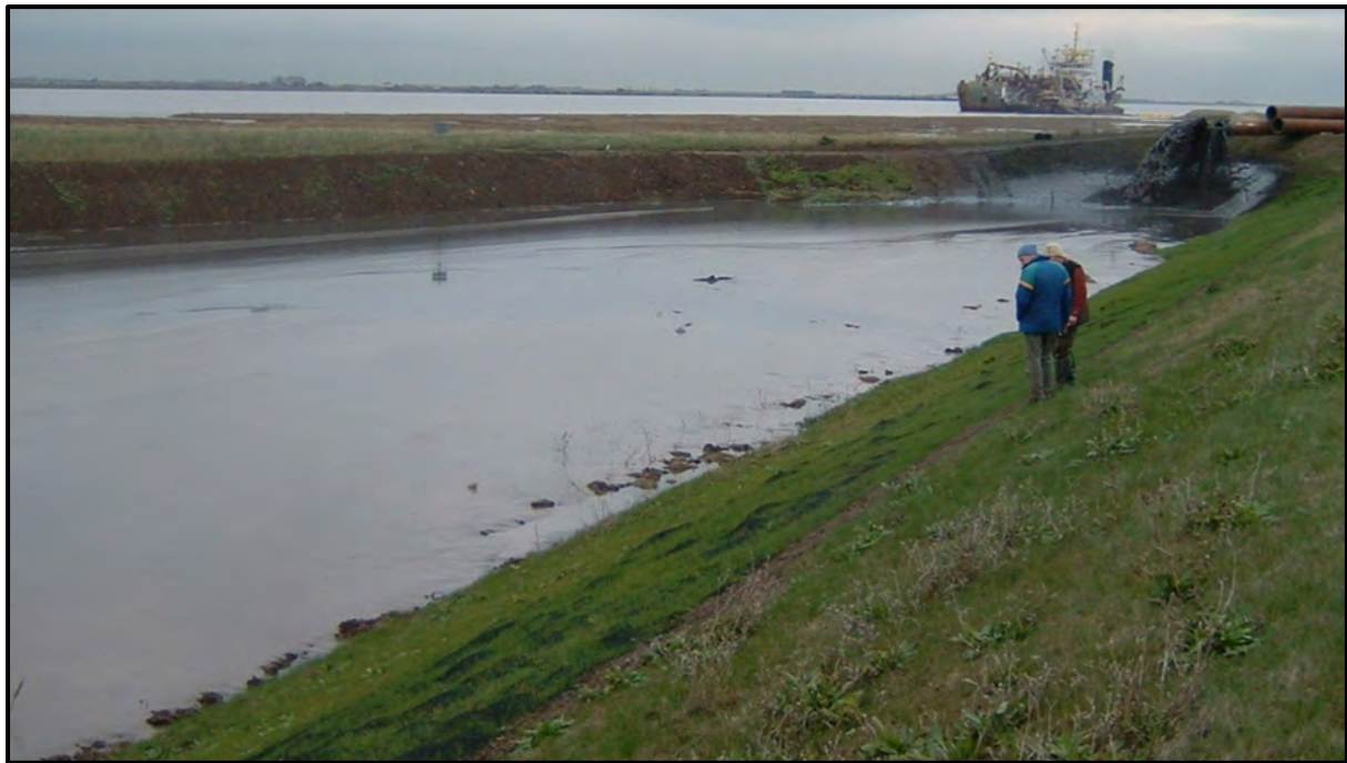
Image 2. Sediment recharge at the Allfleet's Marsh Managed Realignment site
