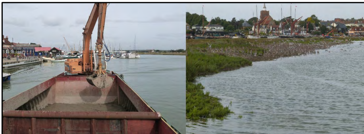
Image 1. Maldon saltings recharge showing barge-mounted excavator and recharge area
