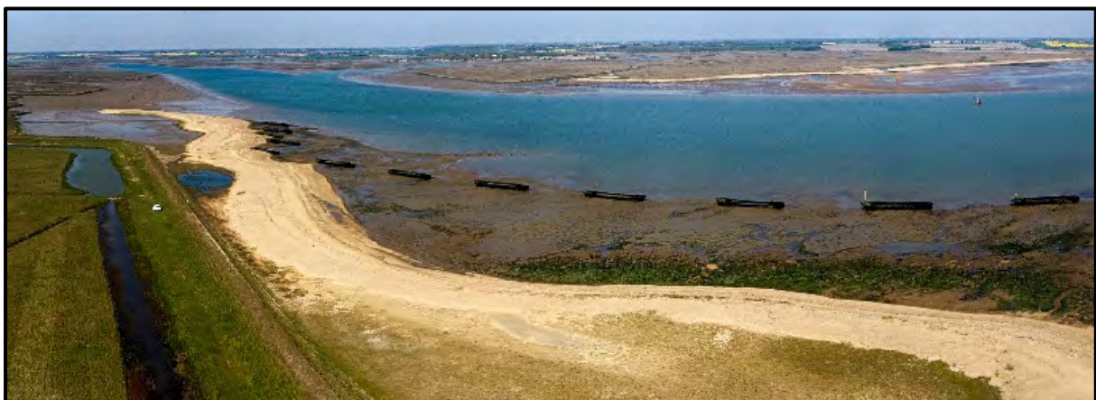
(Jim Pullen UAV Surveys April 2017)
