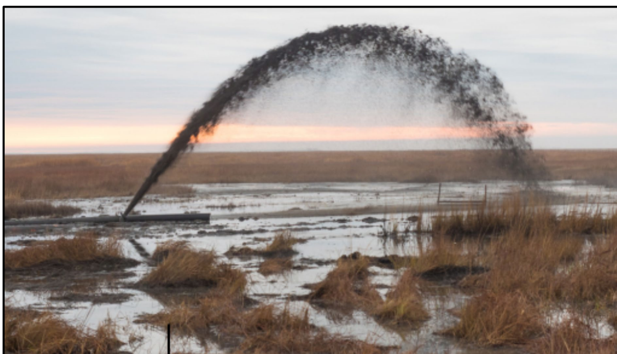
Image 14 Example of 'thin layer deposition' at the US Blackwater National Wildlife Refuge
