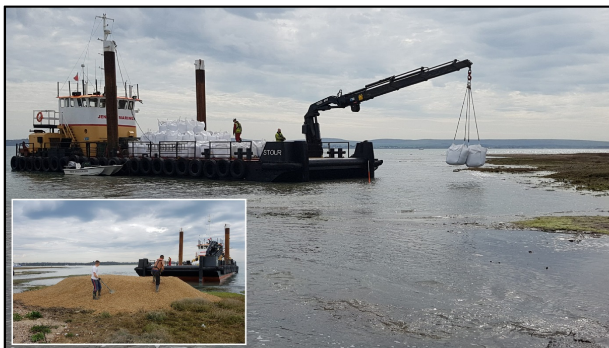
Image B3. Chenier recharge using shingle material at Lyminster River entrance
