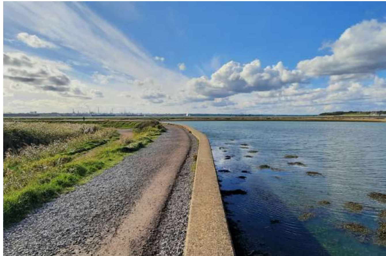
Image of the main embankment at Hook Lake
